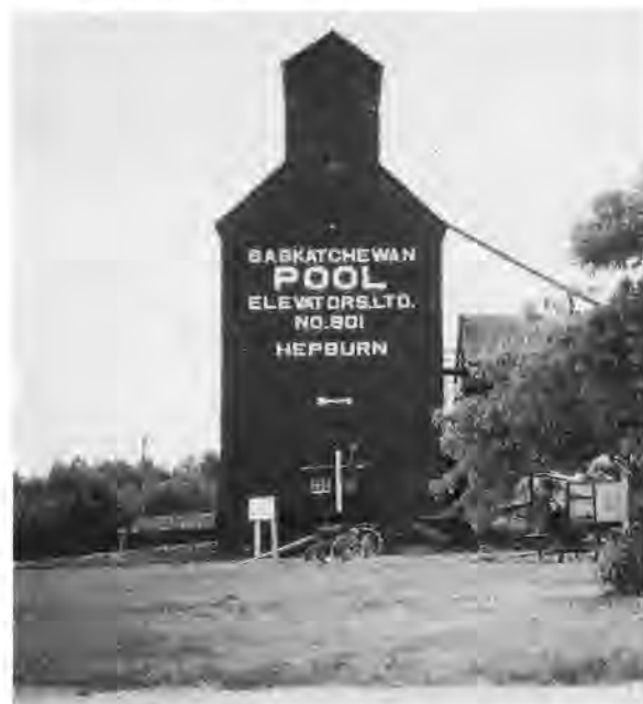
Hepburn Pool Elevator now operated as a Museum.
